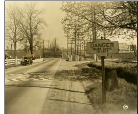
FIGURE 7: ORIGINAL PHOTO OF FRONT-MOUNT “DANGER” SIGN AND POST.
